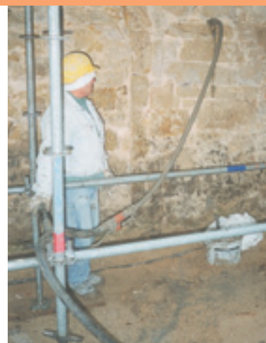
The drill holes for the stainless steel anchors, serving to reinforce the masonry, were mechanically grouted.
