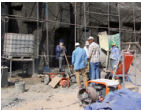
The two PFT ZP 3 S pumps greatly facilitated the construction of artificial rocks.
