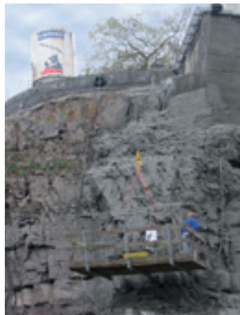
The cliff was stabilized in the wet spraying technique.
