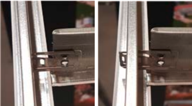
The first 600 mm KDBF cross tee profile should apply as a spacing of 1200 mm on the front .
