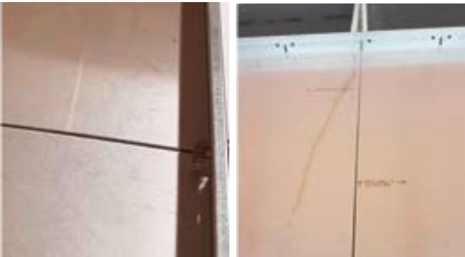
Instead of a cross tee profile, mirror ceiling systems are inserted directly between the T-main runner (butt joined).
