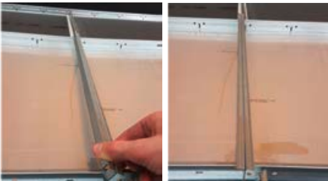
For bracing purposes, the T-main profiles are fixed on the rear with spacer bars.
