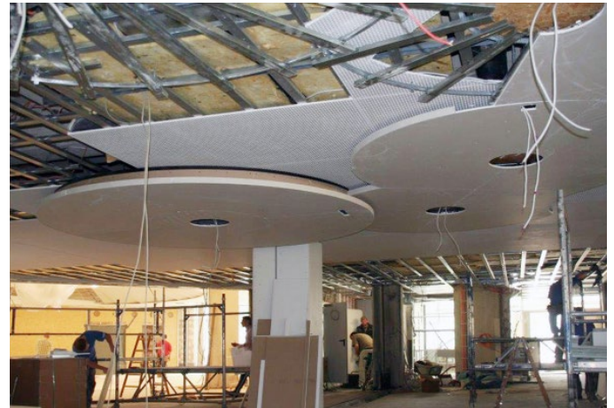
Ceiling construction of the foyer with the three ceiling levels during the building phase. (Photo: Jaeger Ausbau)
