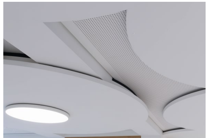
The new ceiling is arranged in three levels in height and cover the relatively low set reinforced concrete beams as well (Photo: Knauf/Clemens Ortmeyer).
