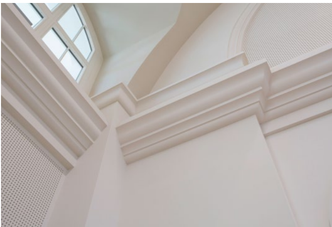
Cornices ex-works: Mitering technology combined with stucco
