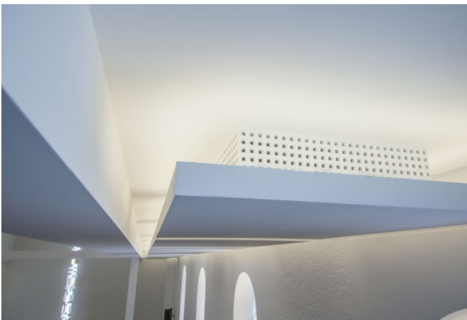
Ceiling canopies made of Knauf Tectopanel acoustic plaster base boards with acoustical plaster absorb the sound in the church.
