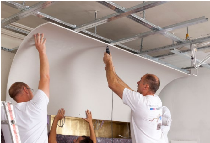
The drywallers manufacture the ceiling canopy above the seating niches in the lounge from prefabricated boards to reduce the assembly time.
