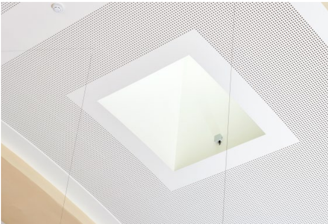
Clad ceiling openings extended right up to the roof covering where a skylight is installed.
