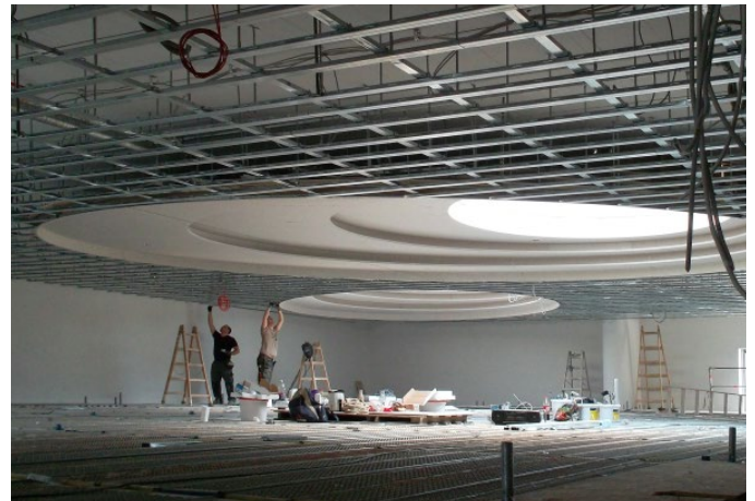
Detail of the ceiling construction in the Max-Planck-Institute. (Photo: Ruben Peter Ausbau GmbH)
