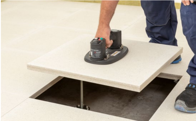
Bild 19: Lifting with vacuum lifting pad
