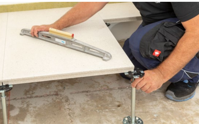
Bild 17: Levelling the raised floor elements
