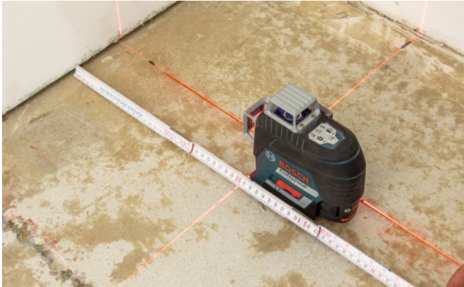
Bild 10: Measuring the wall connection element
