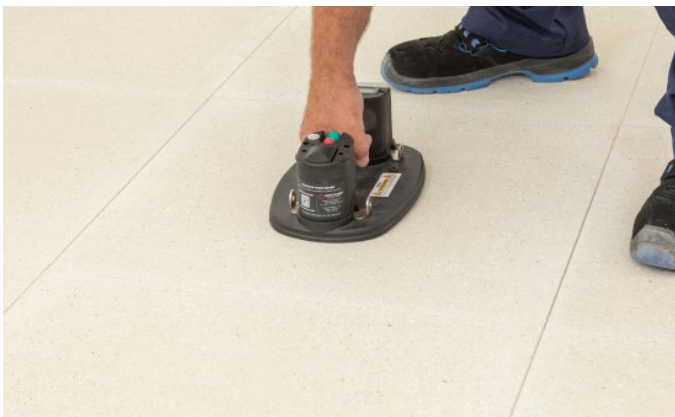
Bild 21: Re-seal raised floor with raised floor element
