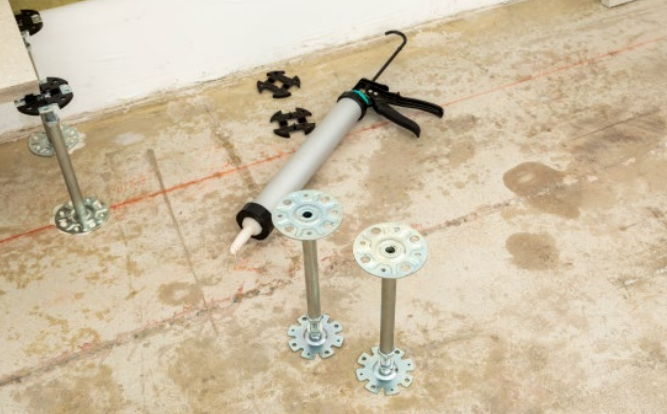
Bild 15: Positioning additional pedestals
