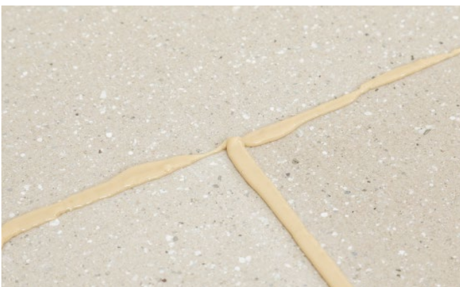
Bild 17: Leaking adhesive indicates sufficient quantity
