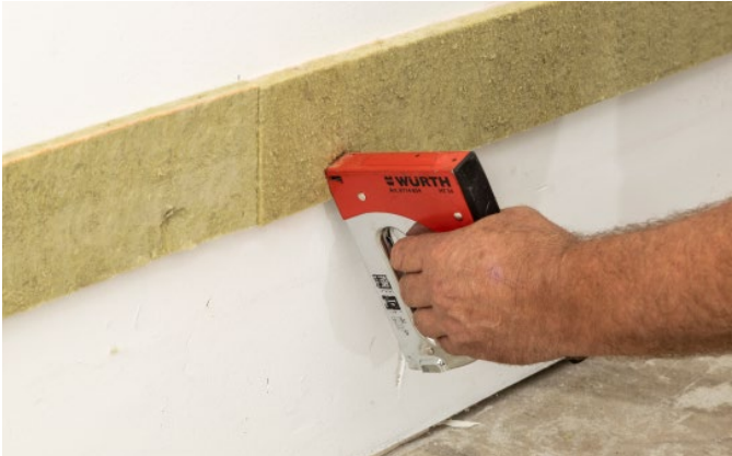
Bild 6: Wall fixing GIFAfloor edge insulation strips
