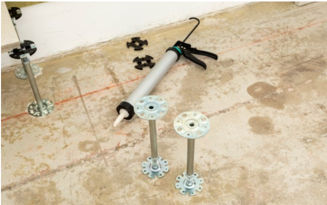
Bild 15: Positioning additional pedestals
