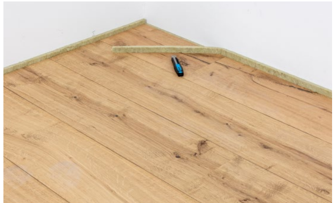
Bild 23: Cut off GIFAfloor edge insulation strips MW flush around the perimeter after laying the top covering
