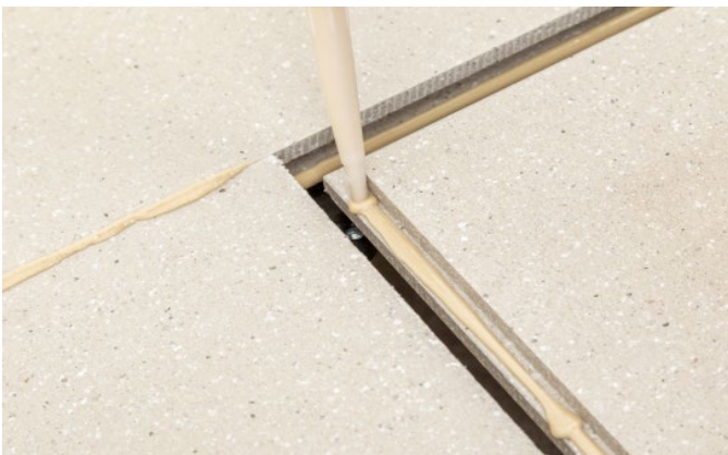
Bild 16: Application of adhesive
