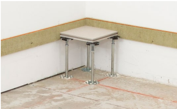
Bild 12: Set up the pedestals and mount them in the wall connection area
