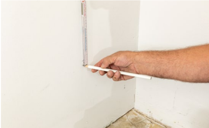
Bild 3: Check and set reference points
