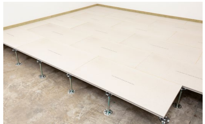
Bild 19: Installation of further hollow floor elements
