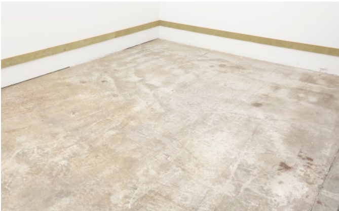
Bild 7: Fasten GIFAfloor edge insulation strip circumferential to wall
