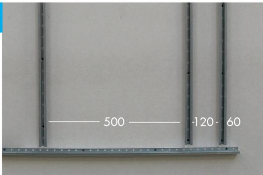
Attach the KDLF 18 mm rails vertically, positioning them directly on the start rail. Install two KDLF 18 mm rails at each end of the wall.
