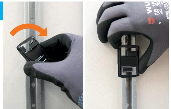
Position the KDLF twist clip at 45° to the KDLF 18 mm rail and twist it in.
