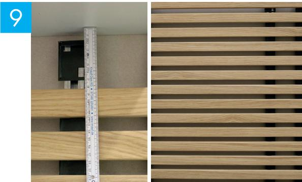
Terminate to ceiling with KDLF end twist clip Minimum spacing to ceiling connection 10 mm.
