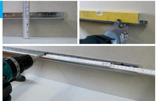
Install the KDLF Start rail horizontal. Spacing between the screws < 125 mm, in dependence on the substrate.
