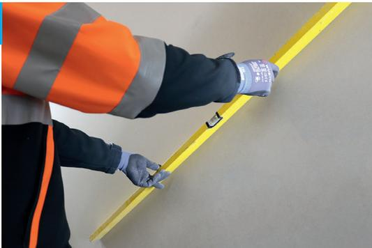
Prepare the substrate, create even surfaces. Optional installation on metal profiles possible.
