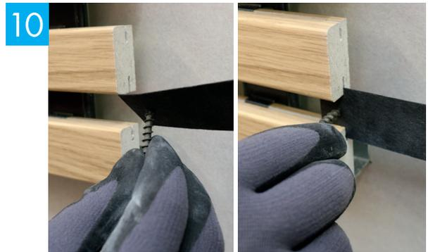
Install KDLF dampers. Tip: A screw inserted into the damper can be used to slide the damper into the grooves.
