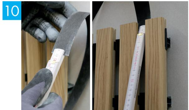
10 Install KDLF dampers. Tip: A yardstick is suitable for moving the damper in the grooves.
