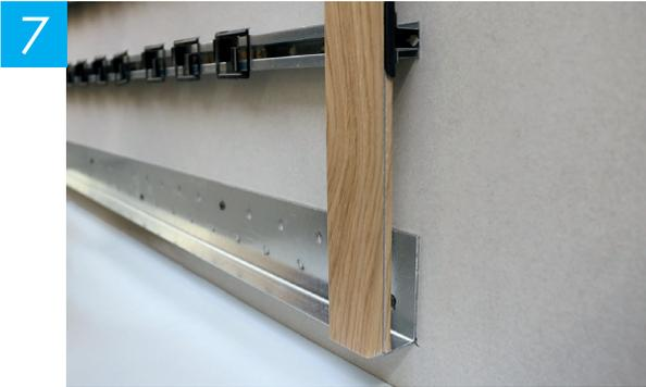
7 Force lock the DESIGNLINE using the KDLF twist clip pushed into place.
