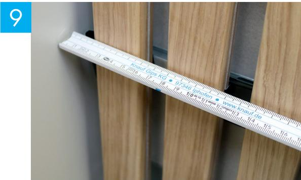
9 Terminate to the side wall with KDLF twist clip by at least 10 mm.
