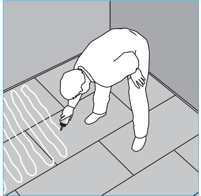
Apply AQUAPANEL® Slot Adhesive (PU) and AQUAPANEL® Joint Adhesive (PU) with gaps of 10cm.
