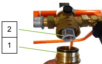
Fig. 49: Strainer screen in pressure reducer
