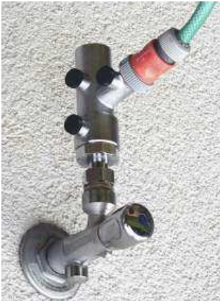
e.g. backflow preventer BA295STN from Honeywell
