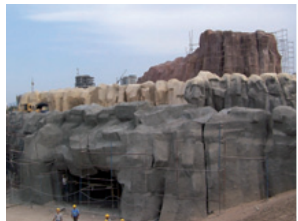
The artificial rock material was applied to the substructure with the aid of the PFT ZP 3 S.
