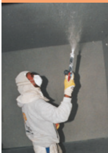
Liquid wood-chip wallpaper was efficiently sprayed onto the ceilings.
