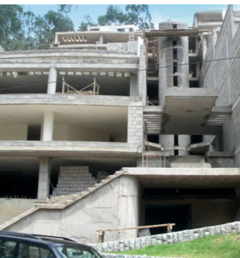
Construction of a villa in the local cement block technique.
