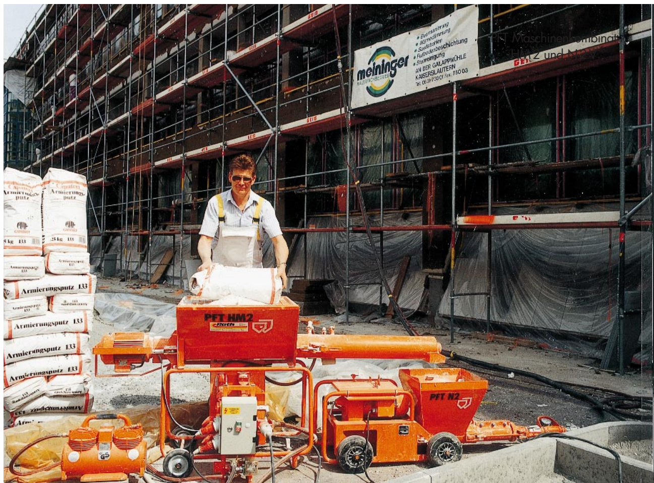
PFT's machine combo of HM2 and N2V keep things in motion, covering a total area of 5000 m 2 with the reinforcement mortar, Capatect 133. Plasterers: Meininger GmbH, Kaiserslautern, Germany.
