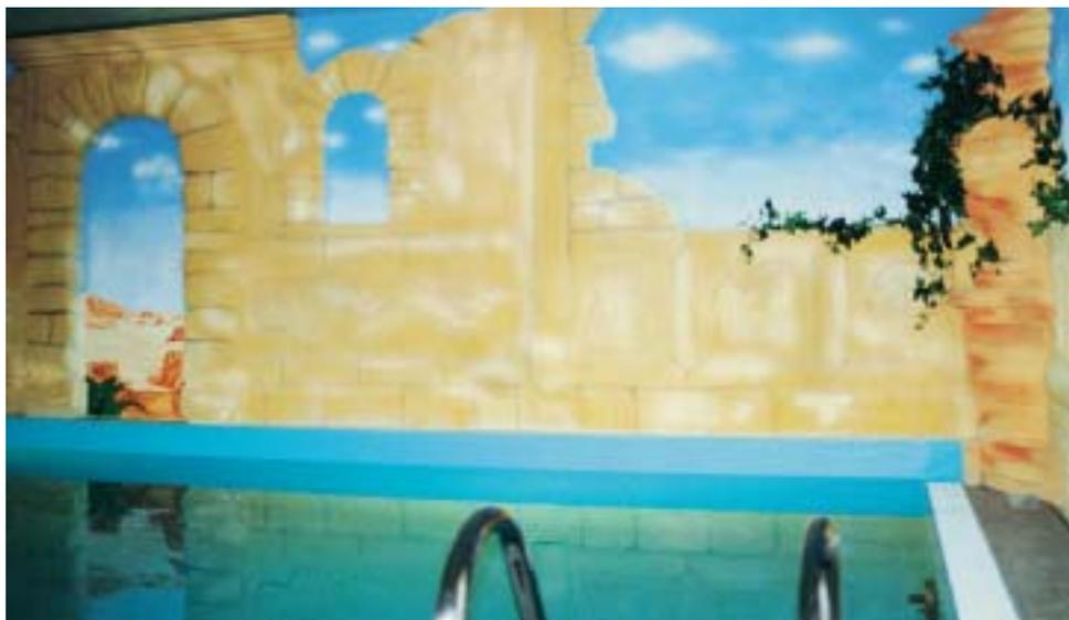
*Not everything that looks like sandstone is really sandstone. Olaf Petersohn models stone relief works like these with the standard nozzle of a PFT SWING. The basic structure is carved out of polystyrene, and the surface is made of reinforcing mortar and filling compound.*
