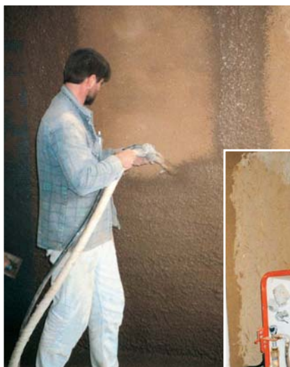
The used clay finish plaster went together well with the PFT equipment and left a neat spray pattern.
