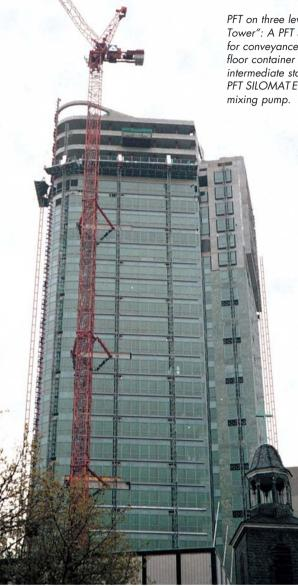
bags". In the "City Tower", however, walls approx. 14,000 m<sup>2</sup> in area were to be plastered with KNAUF MP 75 L. This required approx. 95 tonnes of plaster!
