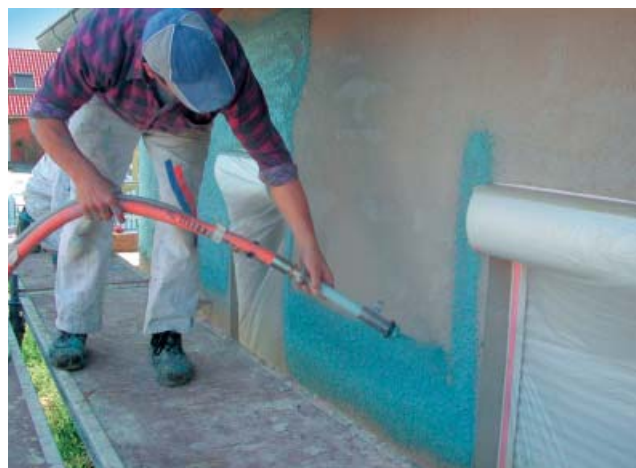
With the aid of a 7.5 metre material hose, the mineral finishing plaster was sprayed onto the wall at a pressure of approx. 8 bar.
