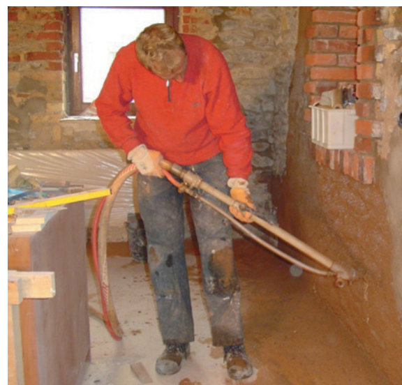
The material is conveyed by the PFT T 10 1.5 screw pump integrated in the PFT ZP 3 long.
