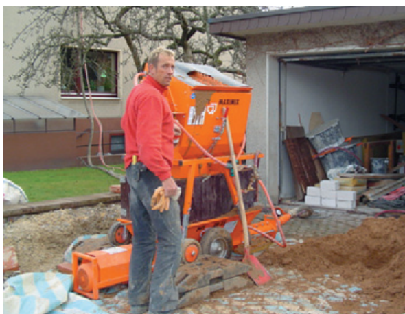
In one-man operation, Frank Siebert can apply large amounts of plaster without constantly having to mix new material.
