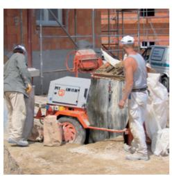
Applying 12,000 m<sup>2</sup> of plaster in six weeks - this can only be accomplished with optimal equipment! The job was done on a piecework basis, and two PFT EM 11 M electric mixing pumps helped to mix and pump the material.
