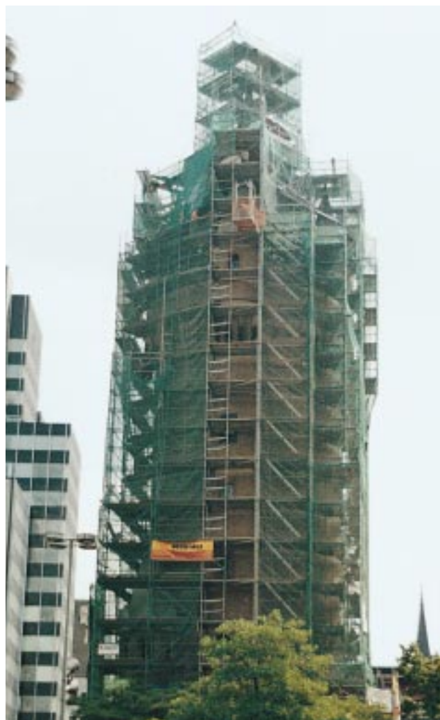
PFT combination-technique SILOMAT, HM 2 and N 2 granted a perfect plastering of the Tower of Eschenheim.
