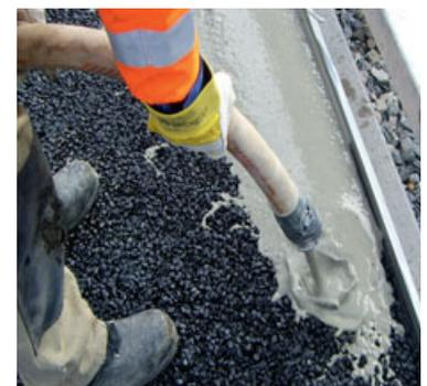
Optimally mixed, the slurry easily flowed into the spaces between the asphalt particles.
