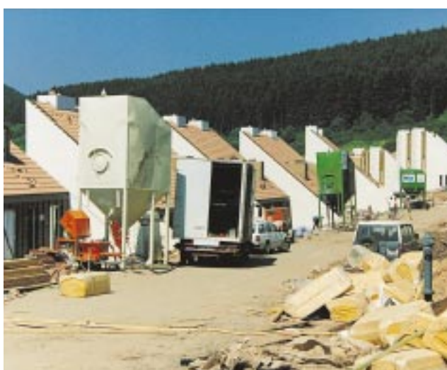
The PFT FMP multifunctional flow screed mixing pump makes it possible to provide screed to 10 to 12 flats a day although the pouring site has to be changed several times.
