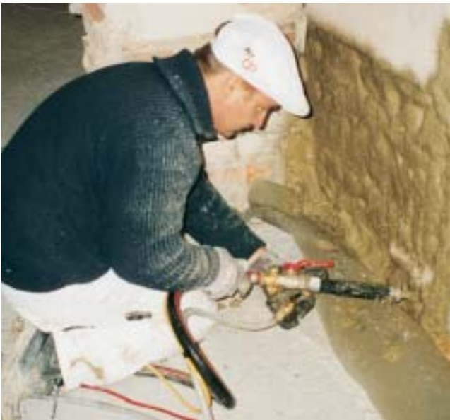
Masonry desalination with „scarificial plaster“. Machine-spraying with a PFT SWING makes this method economical. The applied plaster is knocked off at a later time.
