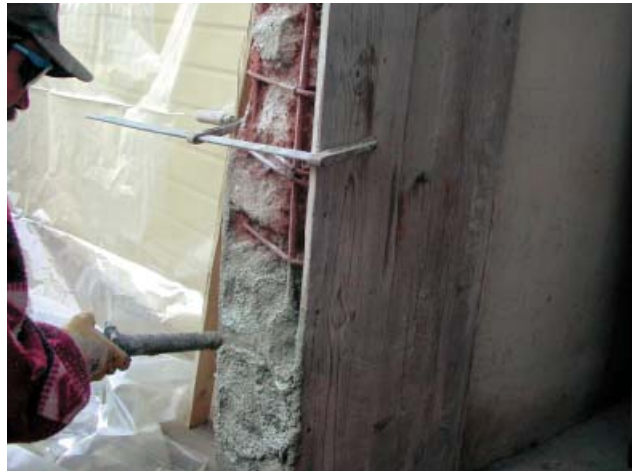
Mixing concrete mortar in a horizontal mixer – supplying it to the PFT N 2 V – feeding it to the mortar pump by means of a worm shaft – and applying it to the wall using a hose and a spray gun: This is the whole secret of SPCC mortar application with the aid of a PFT N 2 V.
