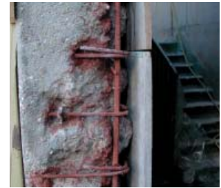
The large concrete spalls had to be "pre-treated" before the actual rehabilitation work could begin: Loose pieces of concrete were removed by sandblasting, a wooden formwork was applied, and the exposed reinforcement received a protective coating.
