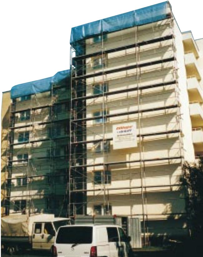
The plaster facade of a house with 24 apartments had been damaged by cracks. Dillinger & Sielaff received the order for its renovation. First of all an armation plaster has been applied within which a crack bridging mesh has been integrated. After the flattening of the armation layer, the final coat was applied. "The most important factor is not the quantity, but regular capacity and quick working" explains Frank Sielaff.
