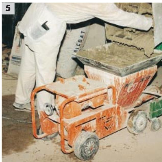
raised to fire resistance class F 90. The usual method of cover roof substratum and steel girders with fire protection plates was ruled out here for reasons related to static characteristics. An additional surface weight of  $40 \text{ kg/m}^2$  would have "overloaded" the old hollow block ceilings.
