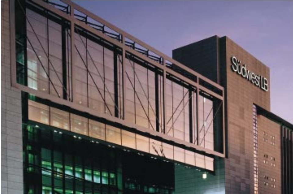
750 t of bed mortar for 6000 m 2 cast stone was mechanically "consumed" in the bank and administration centre of the Südwest LB Stuttgart.
