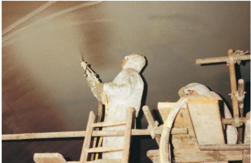
*The good pumpability of the spraying material enabled the use of a 25er mortar hose. The nozzle holder was glad that he had to manipulate less weight, since working over your head is hard enough as it is.*
