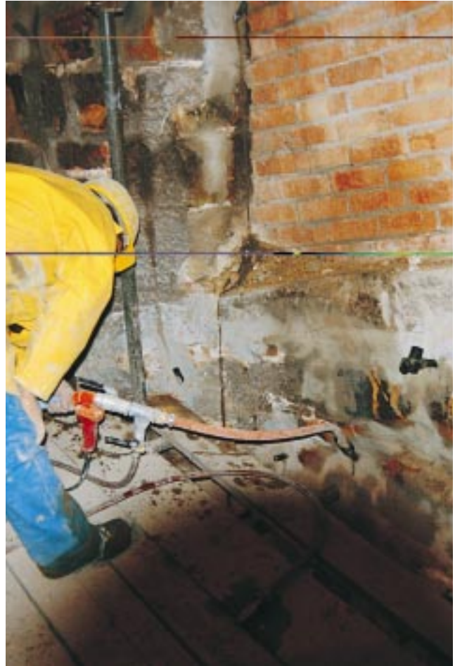
The special PFT injection gun being used to inject mortar.
