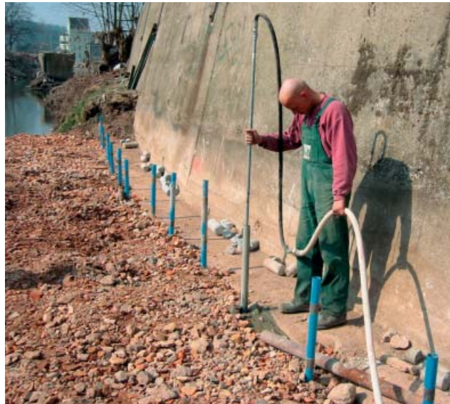
Thanks to the use of an injection lance, the cement suspension flowed even into narrow cavities.
