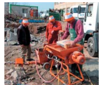
Bag by bag, blast furnace cement was used as a grouting material.
