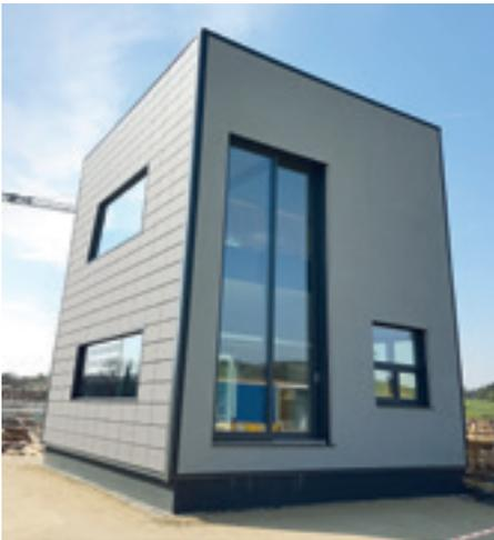
the "Plug & Play" principle. This means that one unit is delivered to the desired location, placed at the correct spot, and then integrated into a building via advanced connecting systems.
