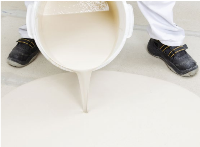
Figure 56: Manual application of Knauf N 410
