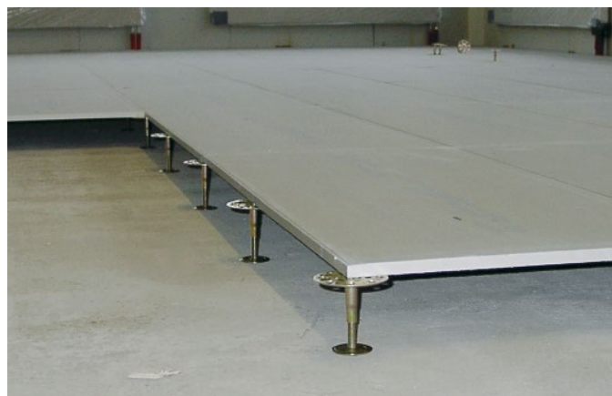
Figure 14: Installation of pedestals and sheathing units
