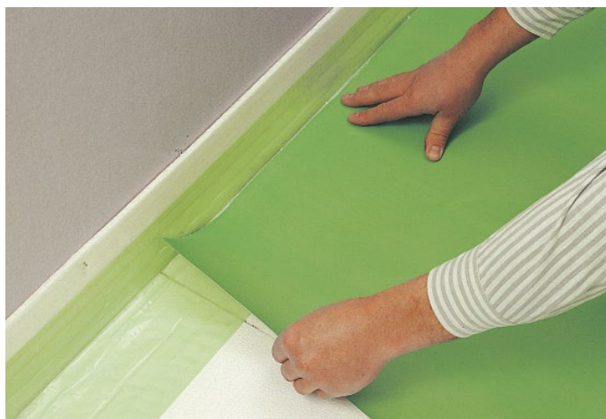
Figure 8: Laying Knauf Schrenzlage synthetic coated kraft paper
