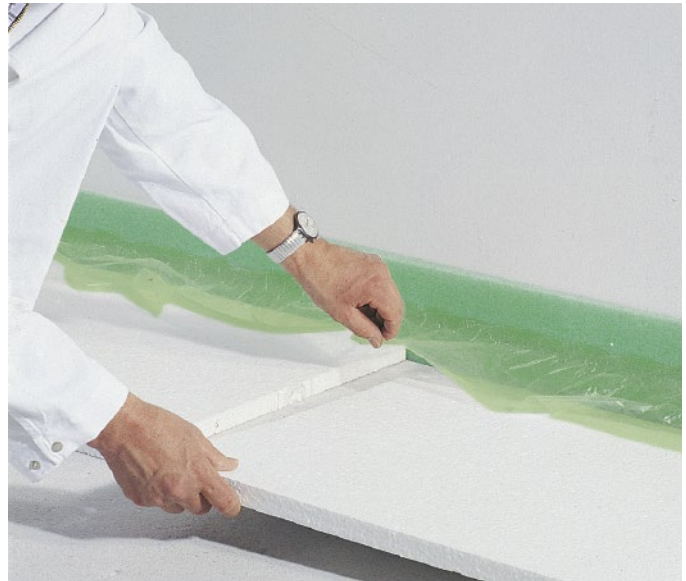
Figure 24: EPS insulation
