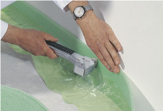
Figure 22: Apply Knauf edge insulation strips with foil (also on pipes, radiators, etc.). Do not staple at screed height.
