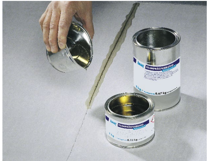
Figure 54: Filling cracks with epoxy resin
