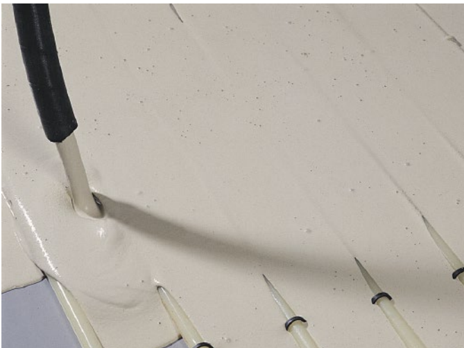
Figure 10: Apply the heated screed
