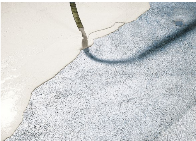
Figure 57: Machine application of Knauf N 410
