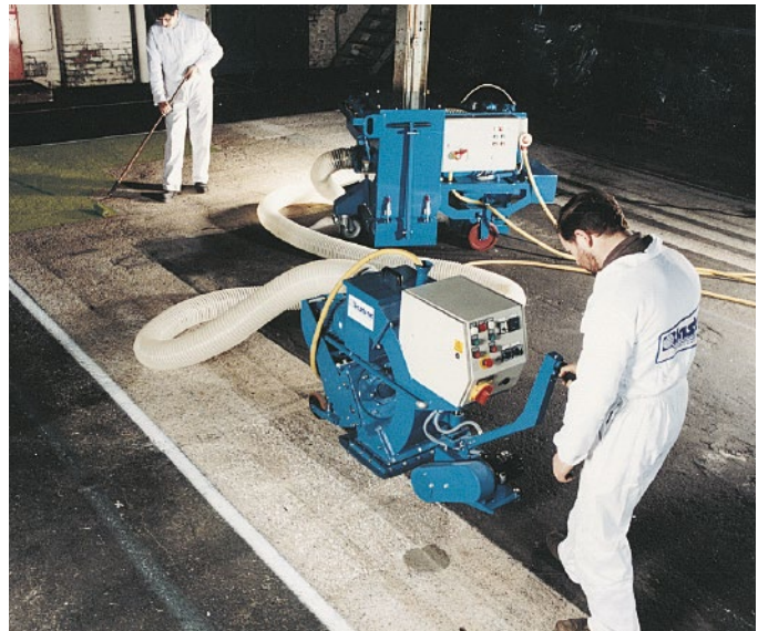
Figure 21: Shot-blasting of the concrete surface to accept a bonded screed
