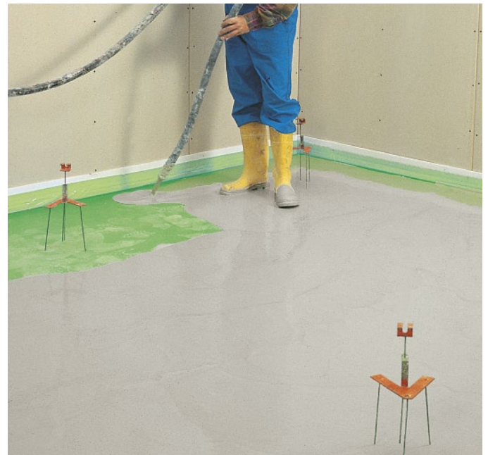
Figure 41: Pouring the screed
