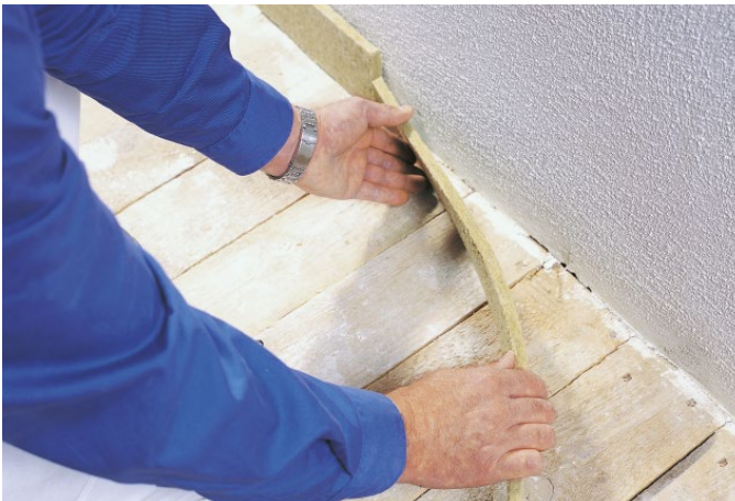
Figure 23: Application of Knauf mineral wool edge insulation strips with fire protection requirements
