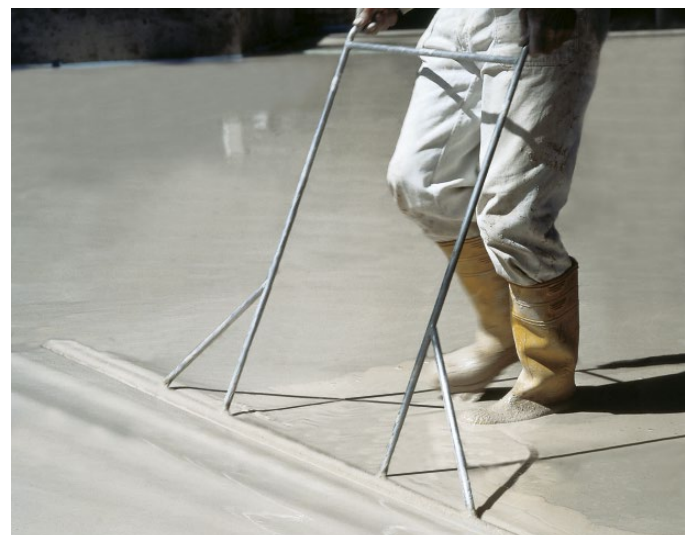
Figure 42: Working with a dappling bar
