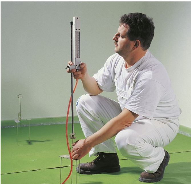
Figure 40: Setting the height with PFT levelling sensors
