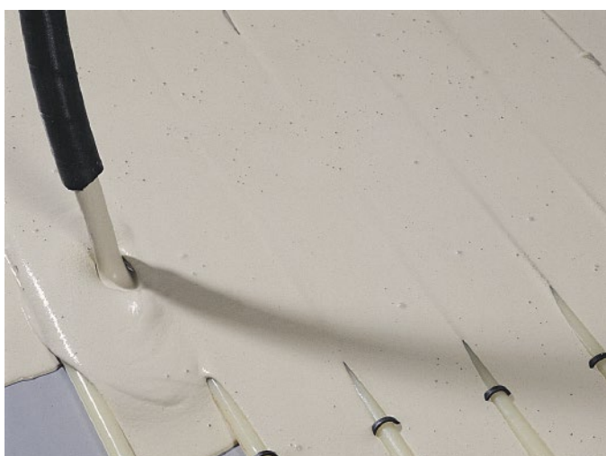
Photo 10: Pose de la chape chauffante
